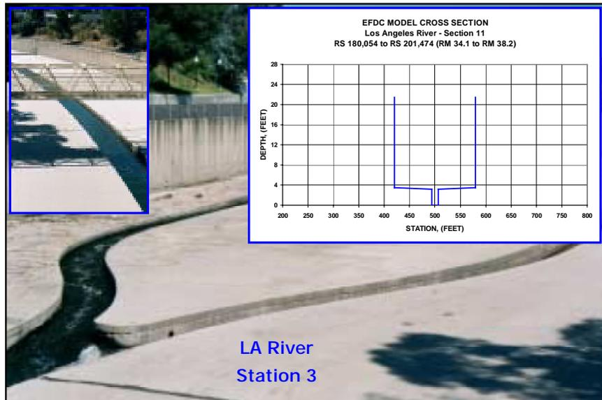
Figure 3: Photo and Cross-Section at LA River Station 3
